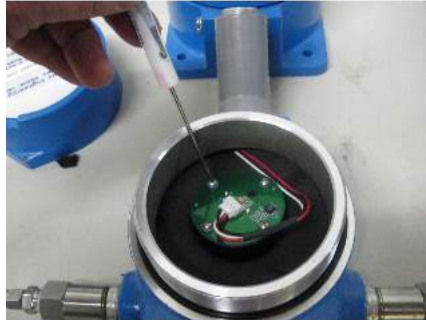
Figure 10: Replaced sensor with all fitting and screws tighten.
